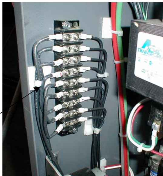
Motor wiring terminal strip (220V Shown)
